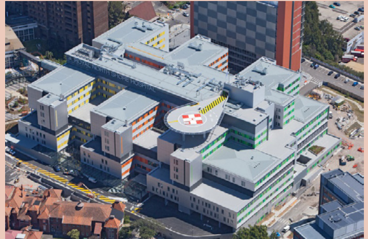
The Acute Services Building at St Leonards (Image courtesy of NSW Health)
